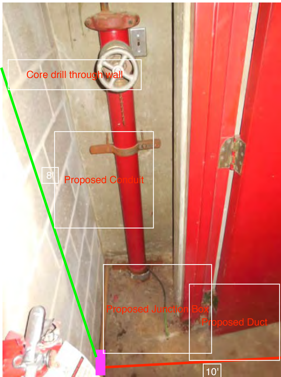
Photo 5 – Proposed Duct / Conduit transition in Room 400
