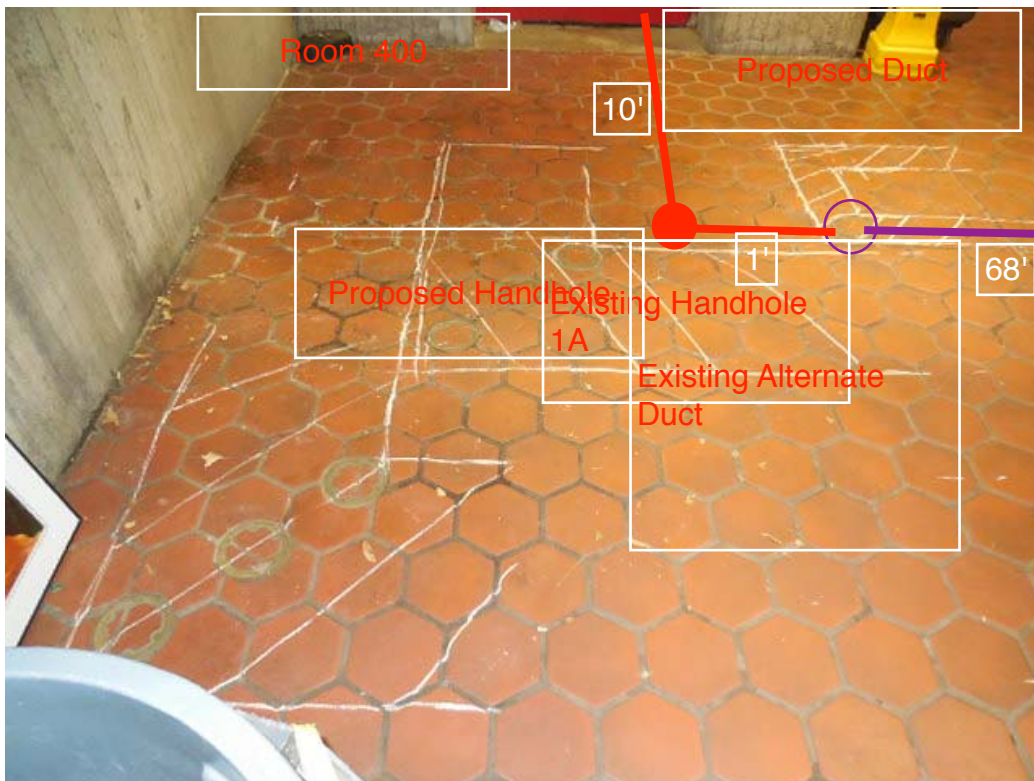
Photo 4 – Existing / Proposed duct layout on mezzanine floor
